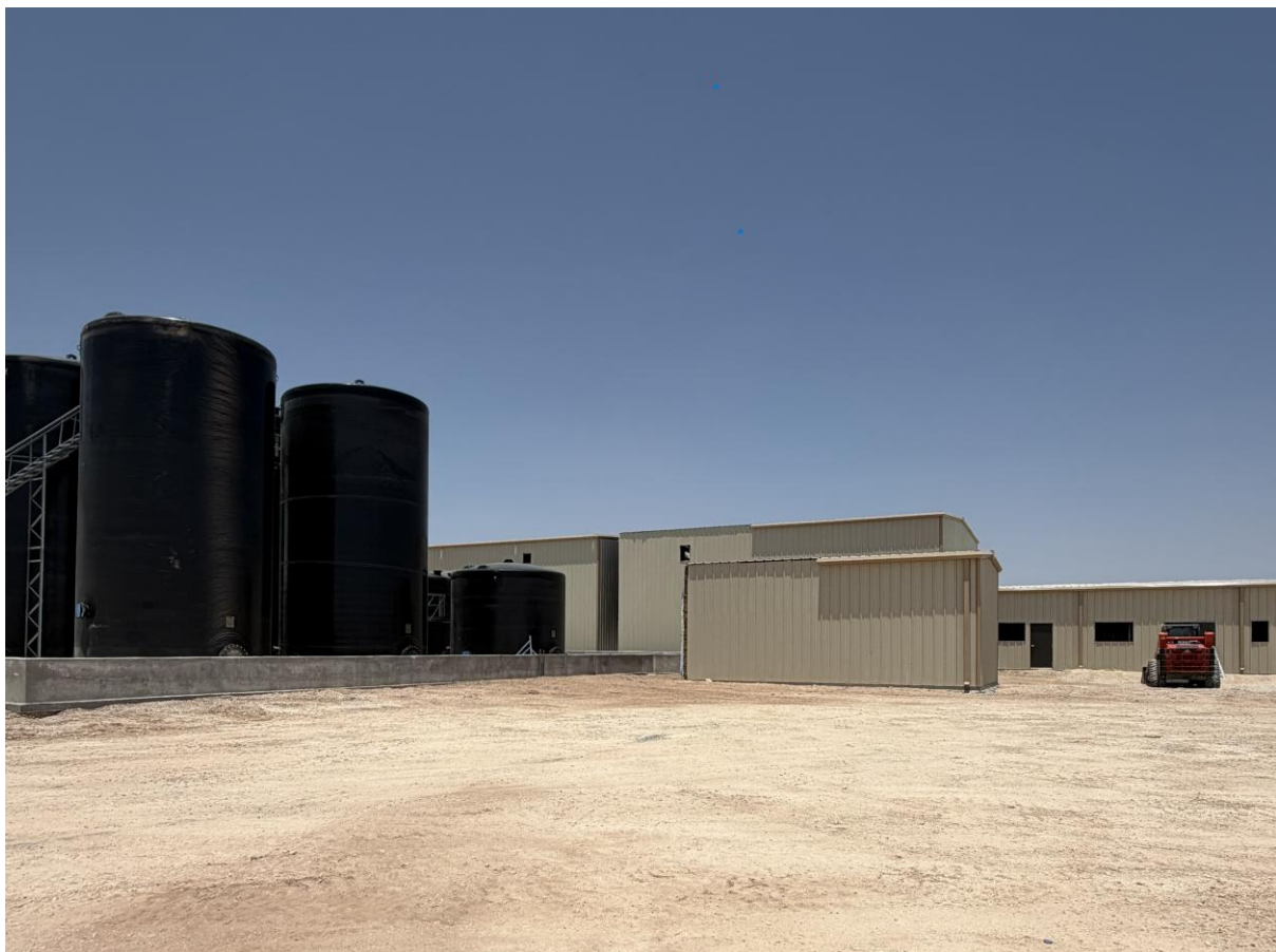
Figure 1: IO#12 construction in the Permian Basin
