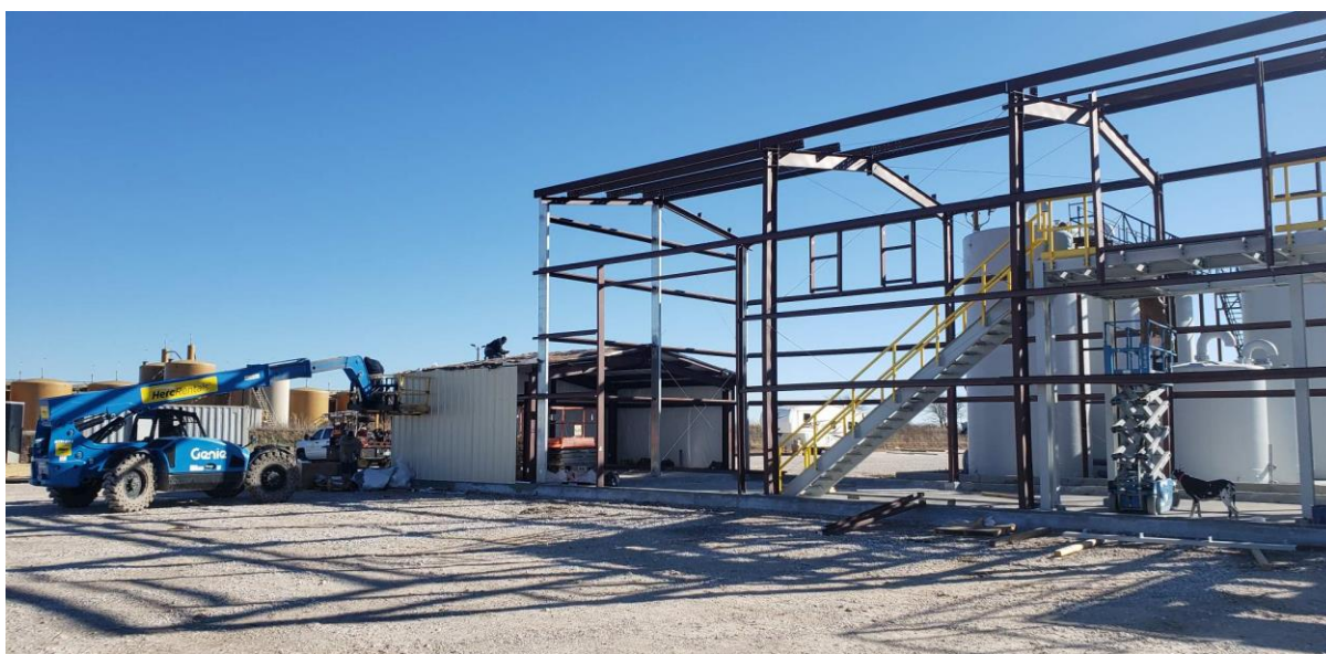
Figure 1. Construction of IO#8 in western Oklahoma
