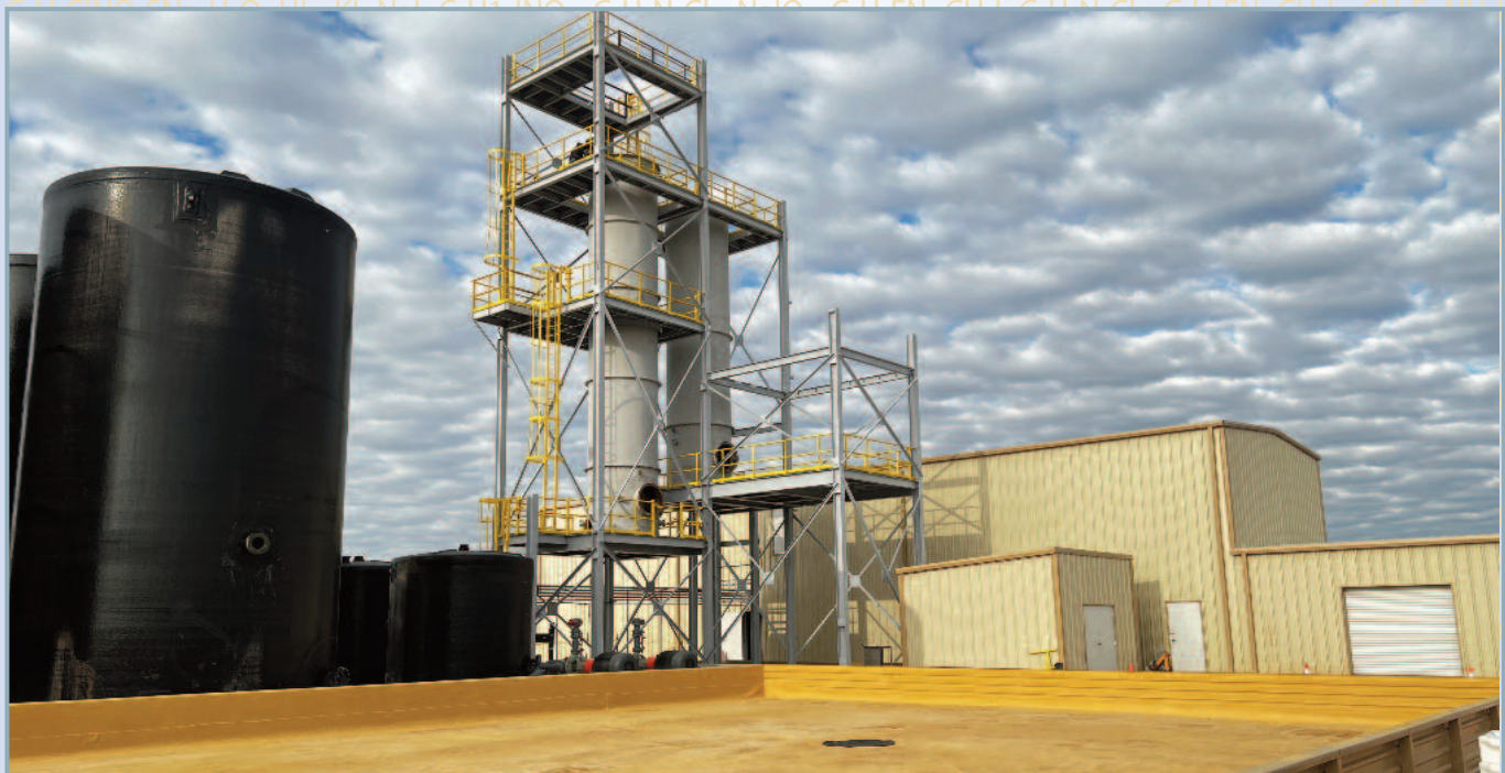
Construction of IOsorb® plant IO#9, Oklahoma USA
