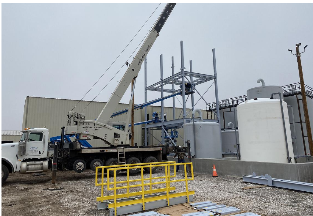
Figure 1. Construction of IO#8 in western Oklahoma
